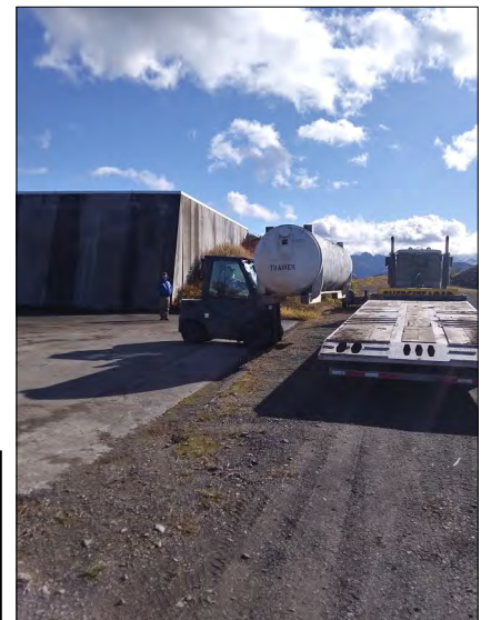
Unloading the missile up at Site Summit. A lot of volunteers and equipment to move the missile. Next step is restoration. (Photo by Greg Durocher)
